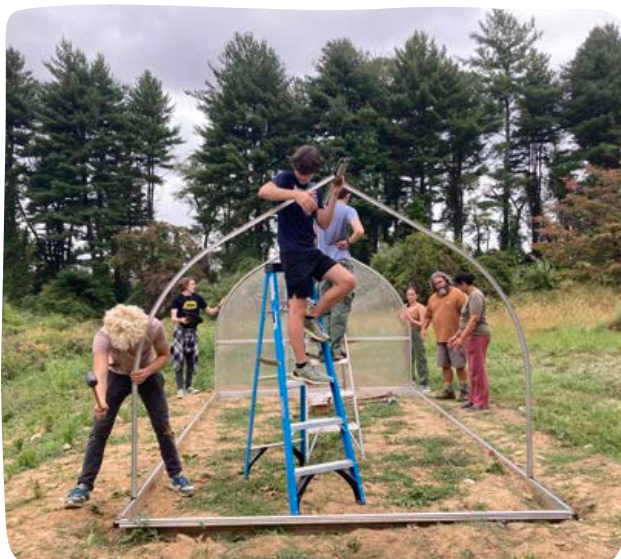
Karl and Locke collaborate to get the front side of the frame assembled and attached to the base, while other SYL members hold the back panel steady.
