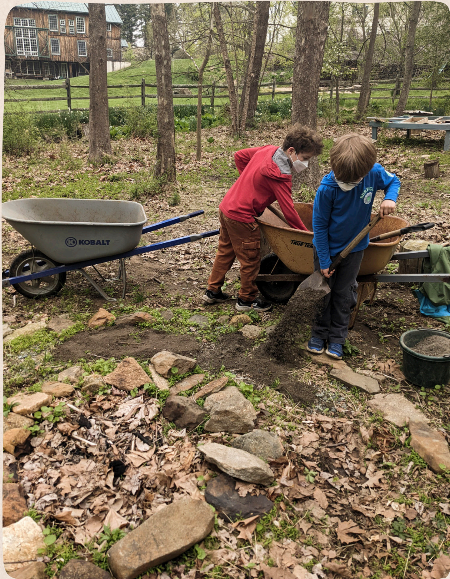
Real work is important in the Open Program. Taran and Brecken work to transfer some of the gravel from the removed Gaga Ball pit to a firepit in our outdoor program space!
